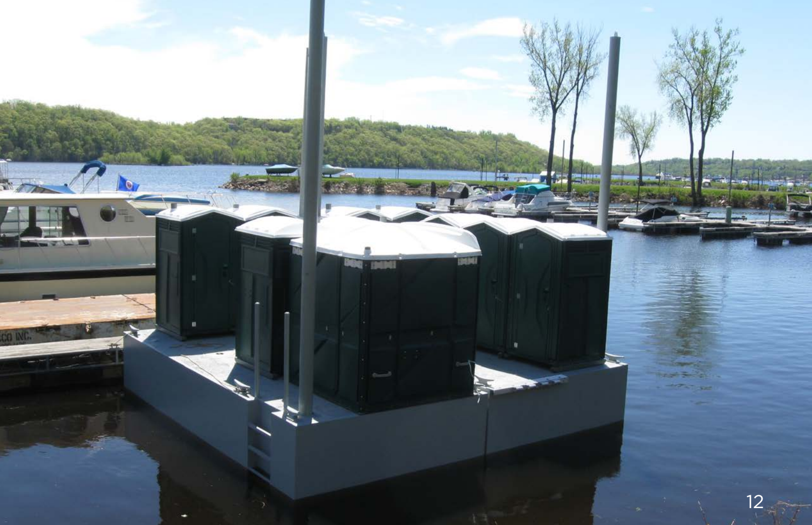
FLOATING WORK PLATFORMS & RESTROOMS
